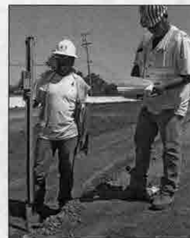
Foreman and eight-year Local 3 member Brian Wilson and Gradesetter Ron Graves, a six-year Local 3 member, check grade on Hwy. 99.
