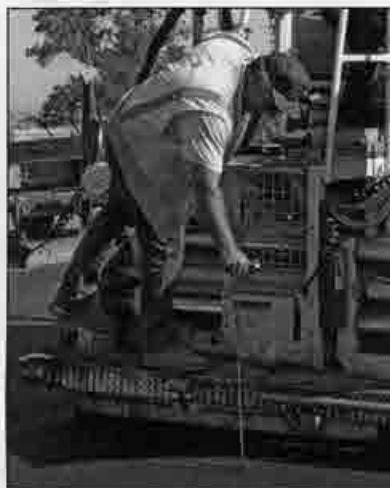
Screedman Kurt Faria, a 19-year Local 3 member, checks compaction of the asphalt on Hwy. 70.
