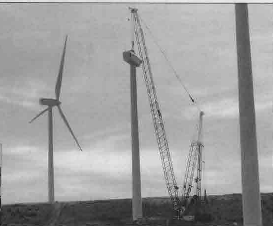
Above: Member Scott Fowden operates a 300-ton Manitowoc M250 with a 275-foot boom to set the windmills into place. At left, from left: H&E Equipment Servicer Tracy Ives and Olsenbeal operators Tyson Allen and Mark Springer work on the Uinta County Wind Farm.
