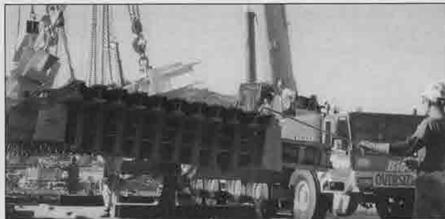
A 200-ton Liebherr Hydro hoists the final 80,000-pound load that will complete the bridge deck.
