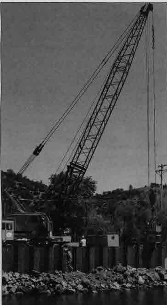
Operating Engineer Mark Powell drives sheet pile at a C.V. Larsen project at the Clearlake Oaks Water Treatment Plant in Clearlake, Calif.
