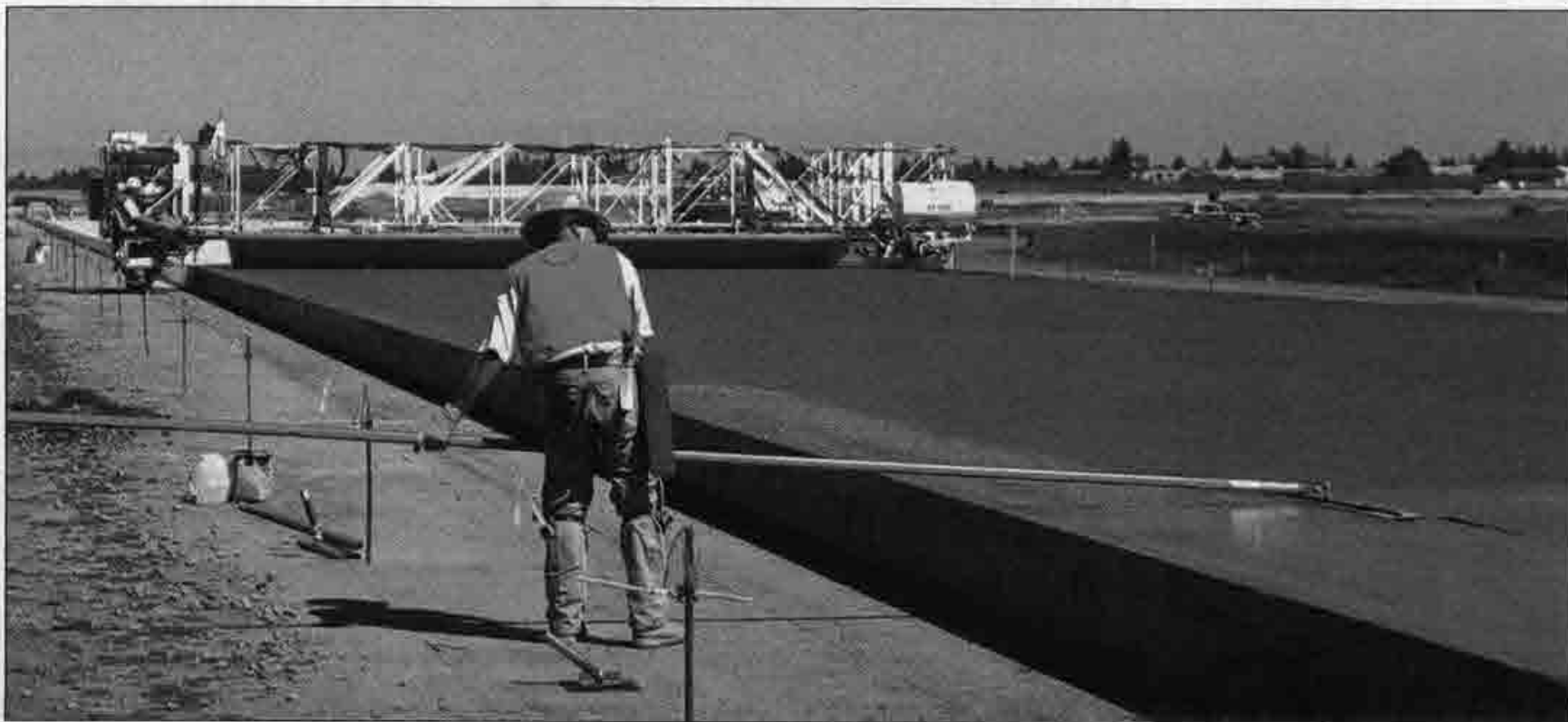
After the concrete is laid, it is smoothed over and sprayed with a curing compound. Gradesetters and gradecheckers ensure that everything is done correctly.
