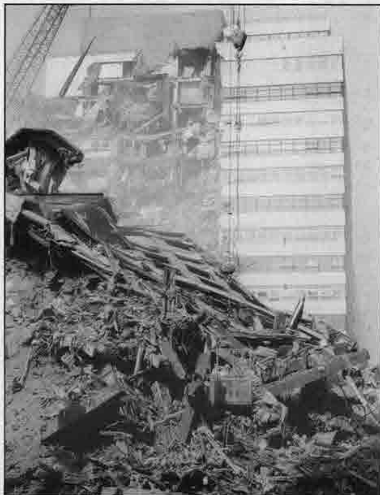
Iron workers in man baskets cutting steel on collapsed WTC 7. WTC 6 in the background.
