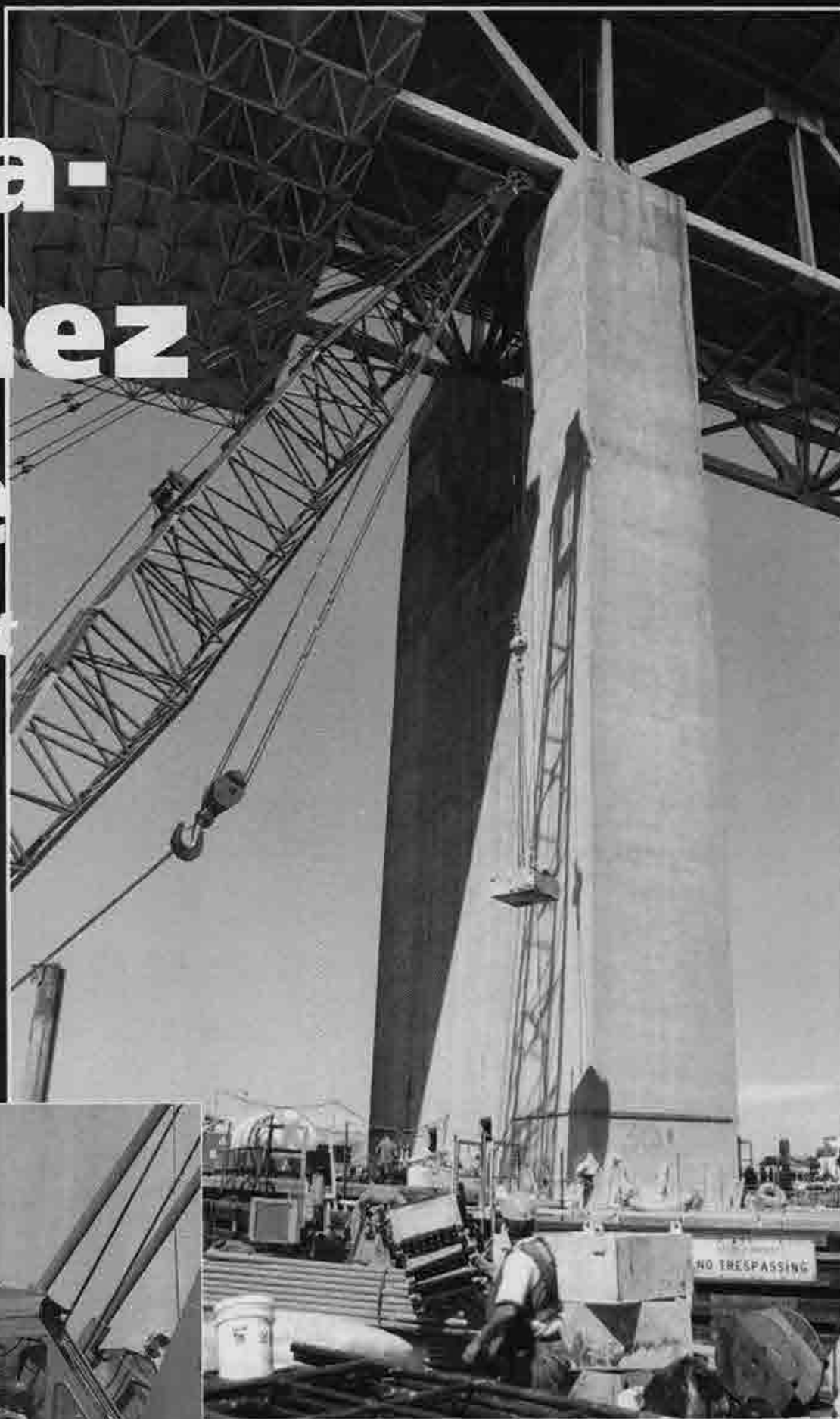
Dale Thomas on a Manitowoc 4000W moves pipe joints from barge to pier area.
