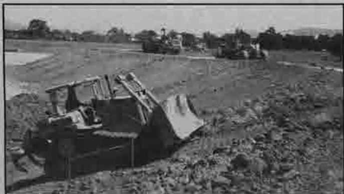
Gary McKay finishes slope inside the pond.
