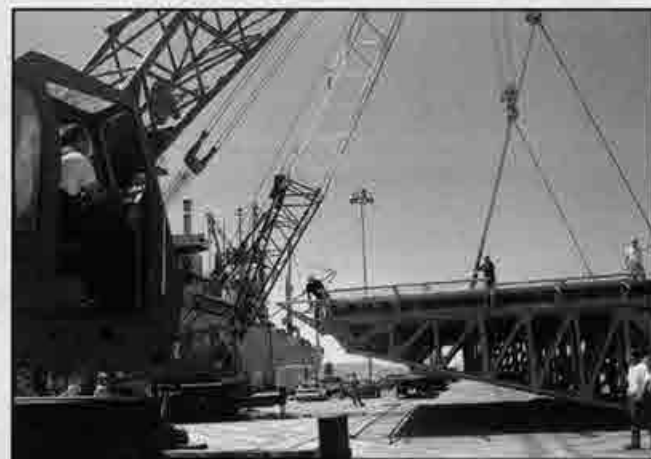
Bill Wentworth, operating near crane, works in tandem with Mark Webster, far crane, to crow-hop the deck toward the edge of the pier.
