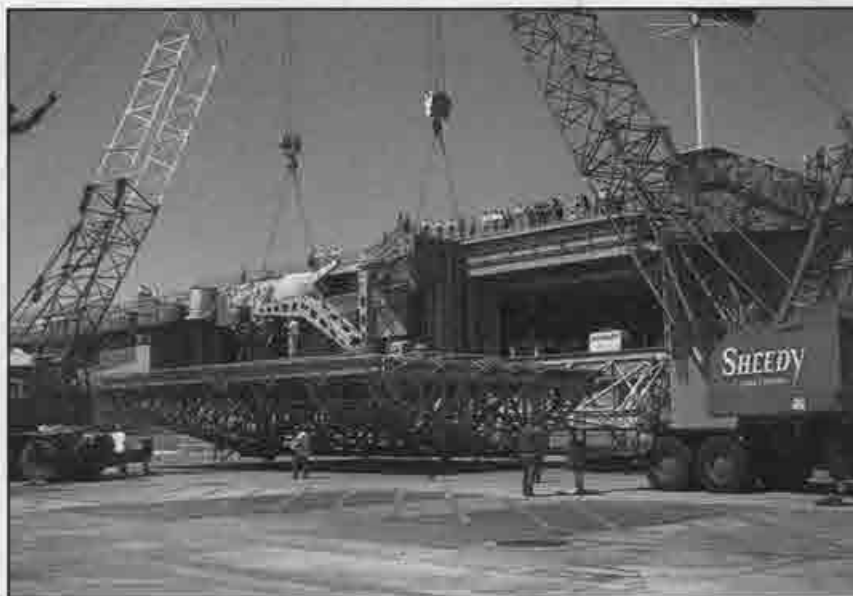
The 52-ton deck is crow-hopped across the pier and into position for the final pick out over the water.
