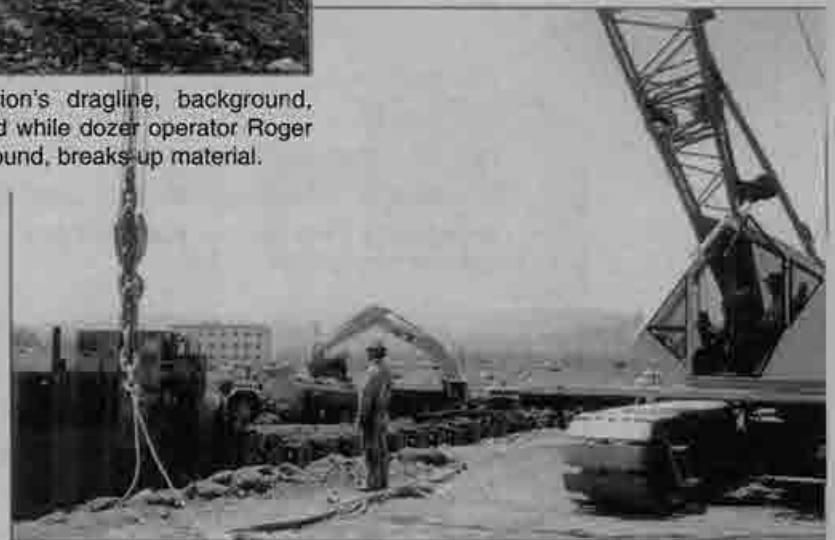
O.C. Jones' heavy equipment digs the marina basin, background, while Dillingham drives sheet piles.
