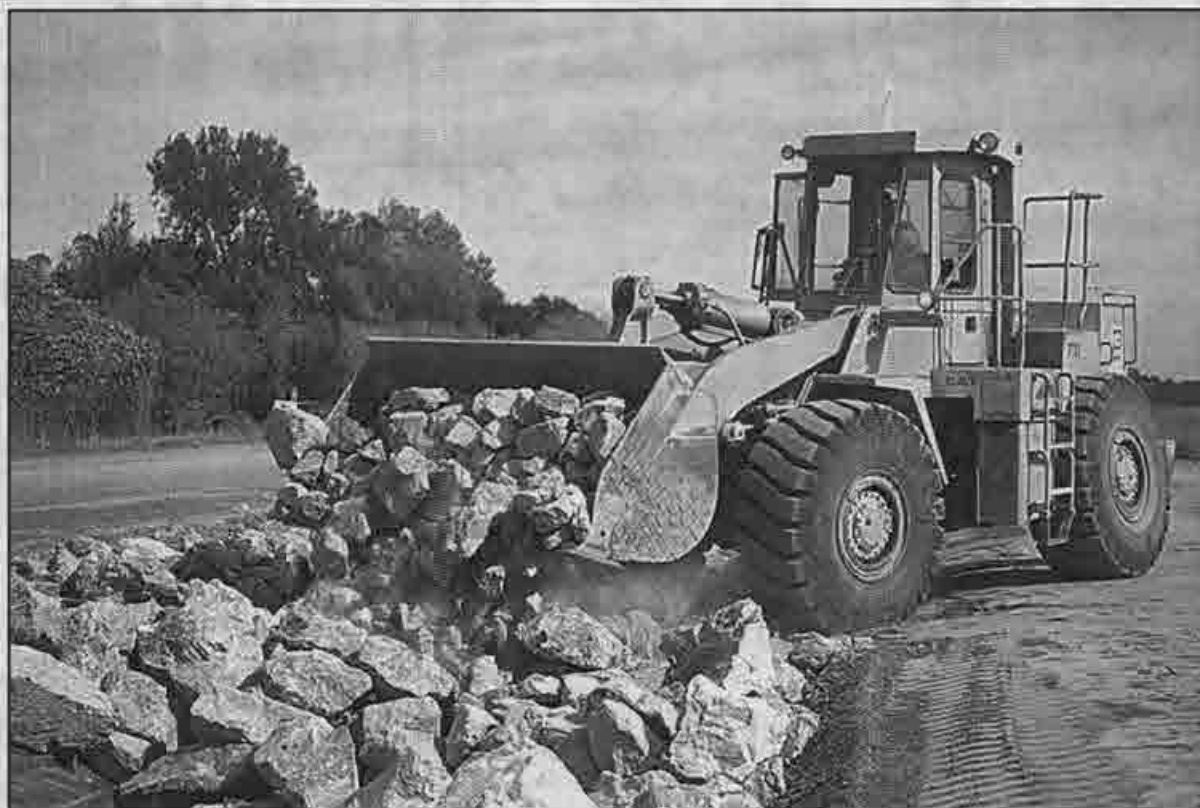
Above: Placing rip-rap is loader operator Jim Marron
