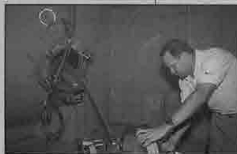
Above: Ed Bowen adjusts probe on 10-D pusher, which is run up into the tubes of steam generators to determine their condition.
