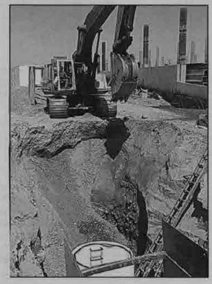
change order for Hazmat remediation work, which entailed pumping the groundwater into a filtering system and decontaminating the soil off site.
