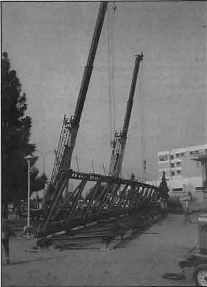
▲ Sheedy crane operators Vince Ellis and Mitch Nevner work together to lift 15,000-pound frames into place.
