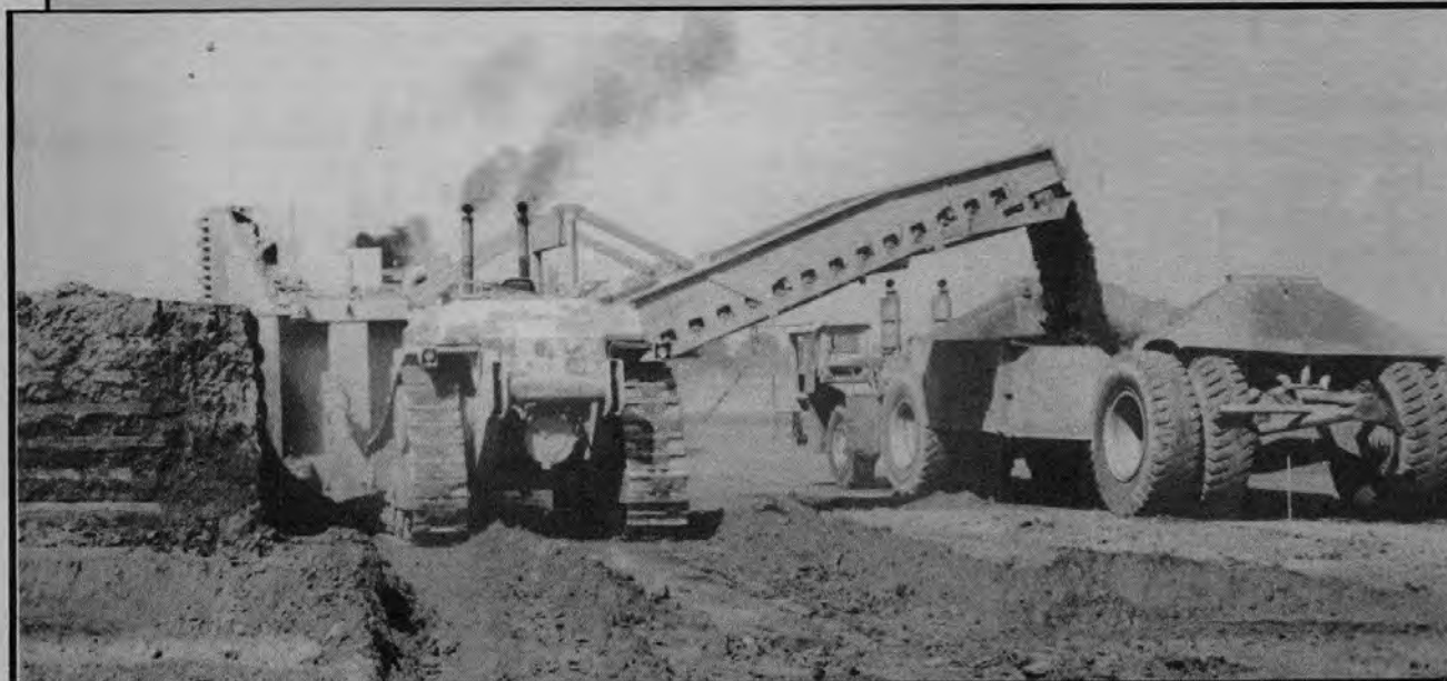
Below: A Holland side loader at the Pup Creek Detention Basin loads this 140-ton haul truck in less than a minute.
