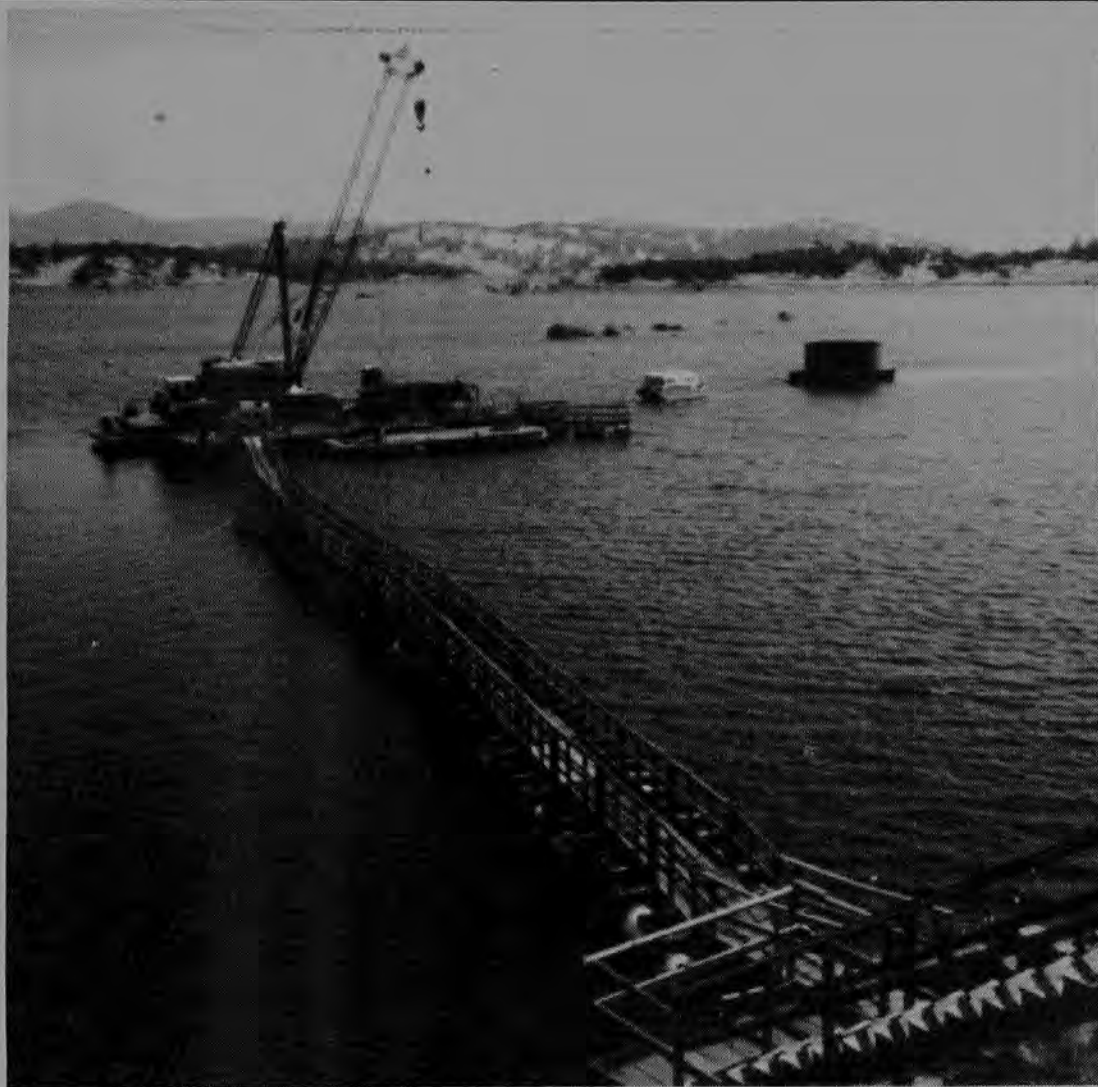
Dwarfed by the Linkbelt crane, Dillingham's "portabarge" tugs a steel shell coffer dam section out to the crane platform. This is one of four 35,000-lb. units to be used in building the coffer dam.
