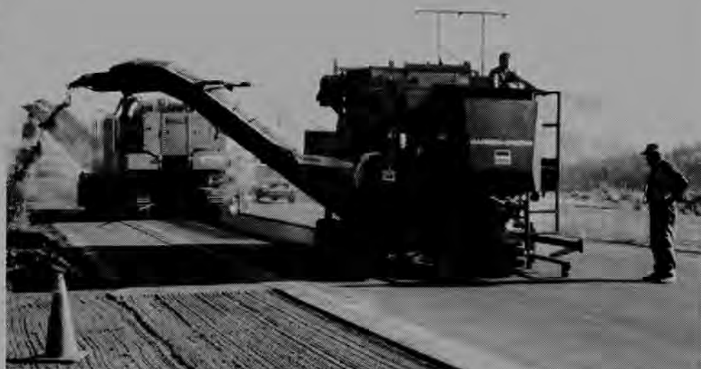
Las Vegas Paving does surface grinding for general contractor Helms Construction on an eight-mile overlay job on I-80 west of Reno.
