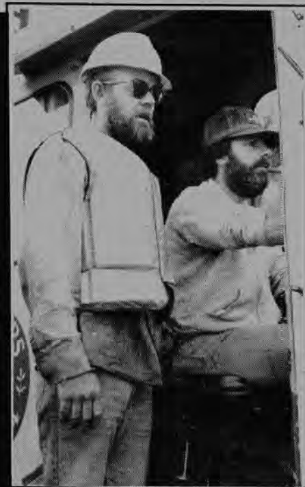
Oiler Tom Smith and operator Bob Stafani work one of the two track-mounted 3900 Manitowoc cranes (right).
