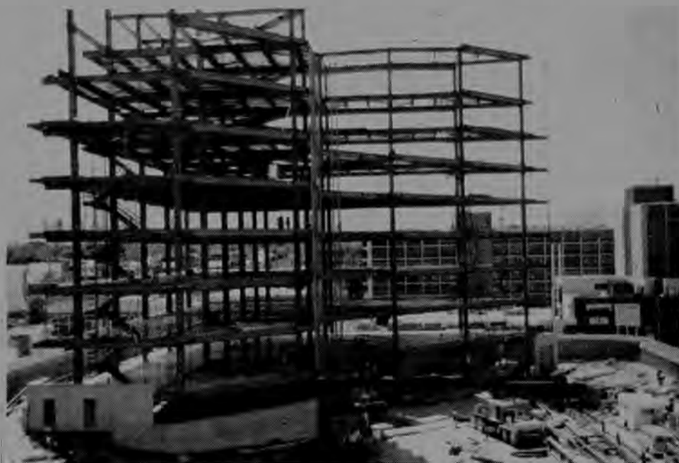
Pictured above is the new Sierra Arts Building currently being built by McKenzie Construction Co. in Reno, Nevada.
