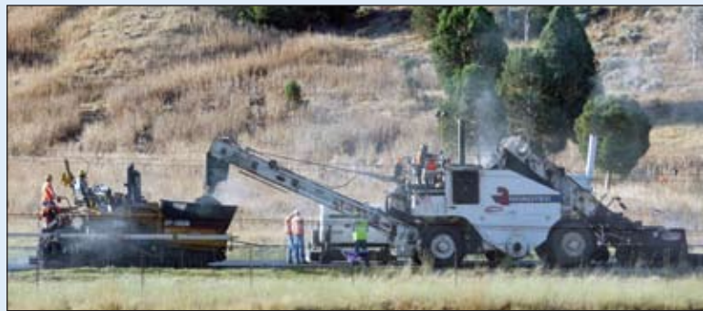
Paver Operator Brian Braithwaite and Shuttle Buggy Operator Chad Vanpatten pave I-80 in Utah.
