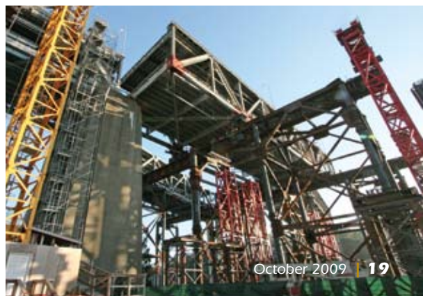
The more than 3,300-ton section as seen from below at 6:58 p.m. Sept. 4, during the bridge roll-out. For more photos, visit oe3.org .
