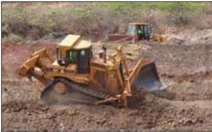
D9 Dozer Operator Justin Johansen cuts the slope at Aliamanu Crater for Delta Construction .
