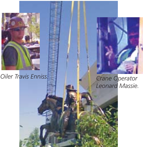
Bragg Crane uses a 300-ton Linkbelt with 310 feet of boom to place a brass statue of a Pony Express rider in the middle of Legends Mall.
