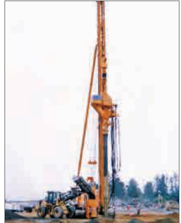
Operator Steve Clark feeds the hopper on the rock column machine in Eureka.
