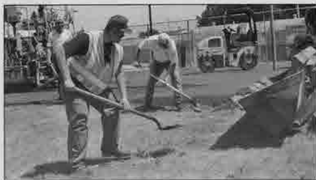
Delta Construction's crew works to lay asphalt on the basketball court.
