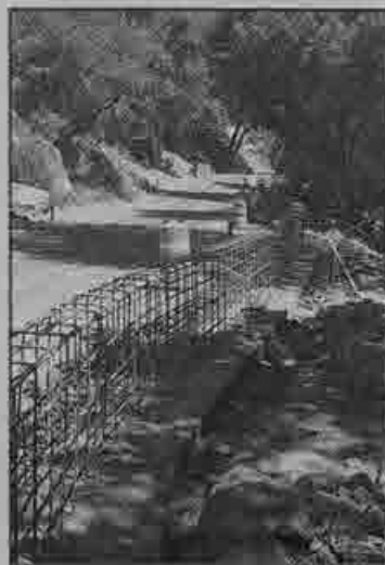
Rebar for new guard wall along Hwy. 140.
