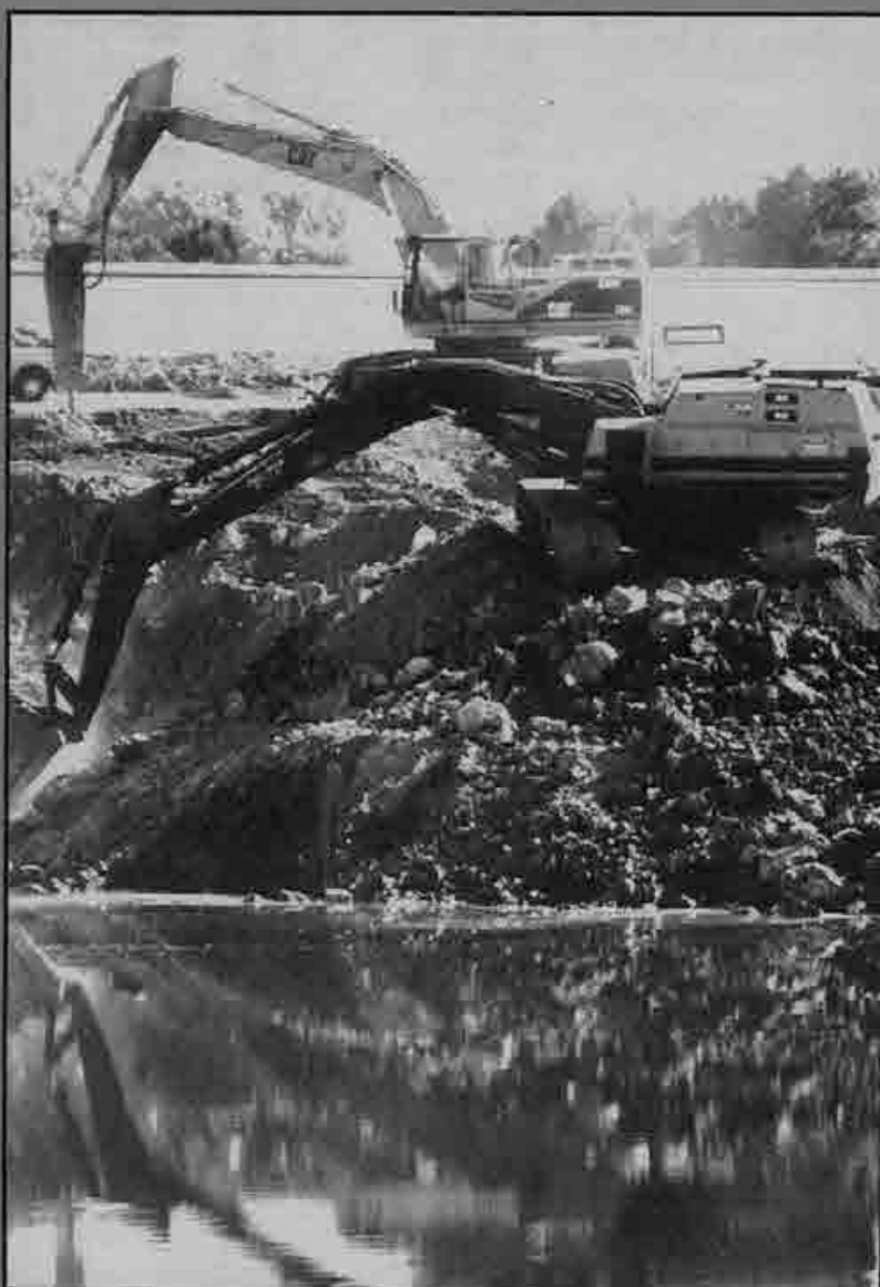
T.W. Construction's Operating Engineers stabilize the sides of one of the pits.
