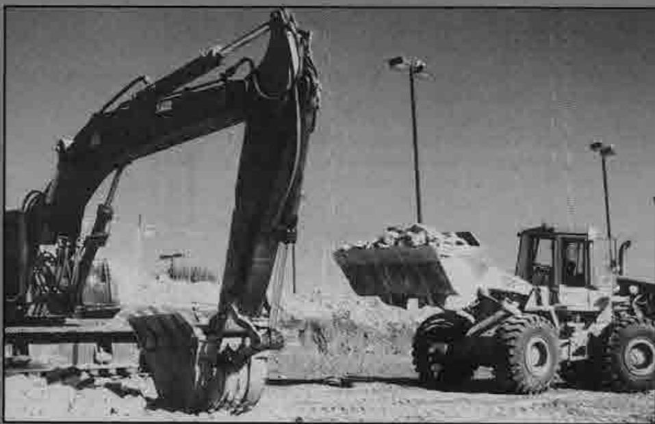
Loader operator Gary Rose feeds rip-rap to excavator operator Ken Julian
