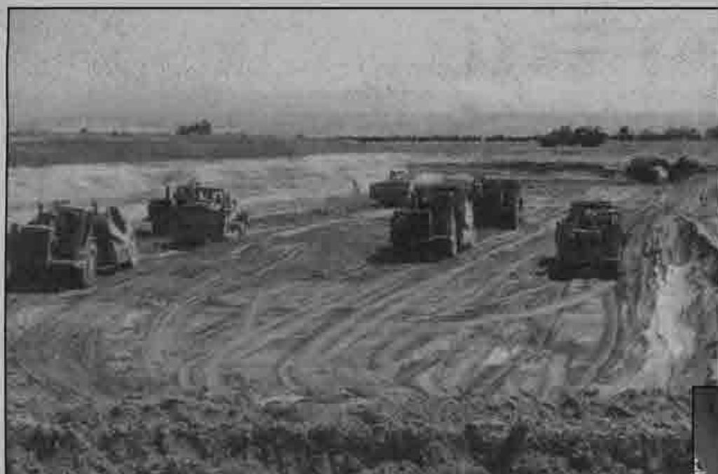
◀ American Paving's scraper crew perform over-excavation down 20 feet to make the soil suitable for construction.
