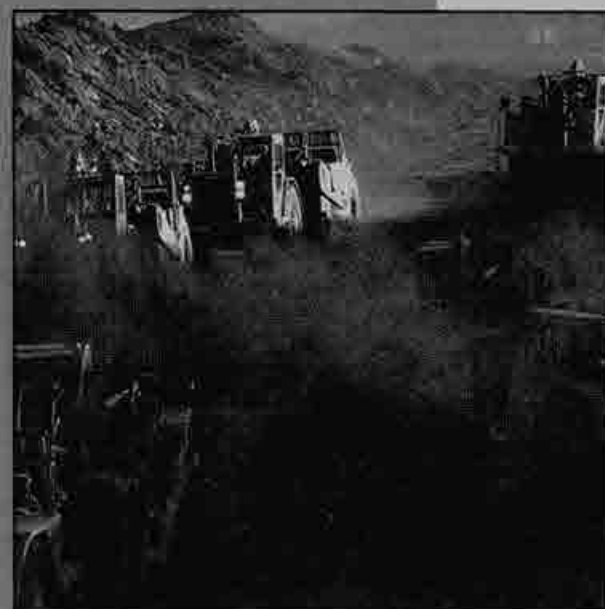
➤ To move the required 3 million yards in 30 days, these scraper hands worked six and seven 10-hour shifts per week.
