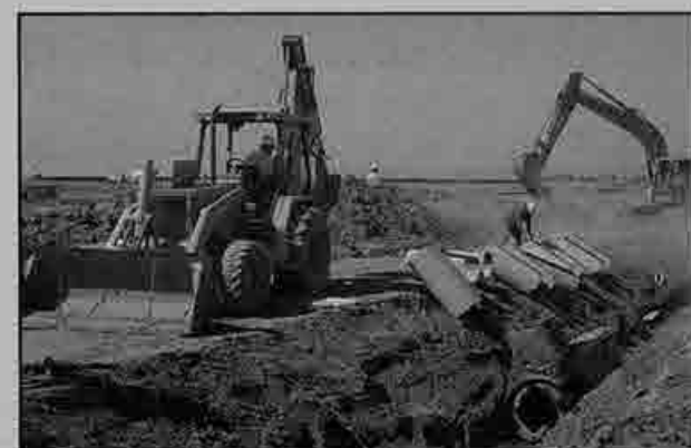
➤ Subcontractor Stoneridge Construction installs 30-inch and 60-inch storm drains.
