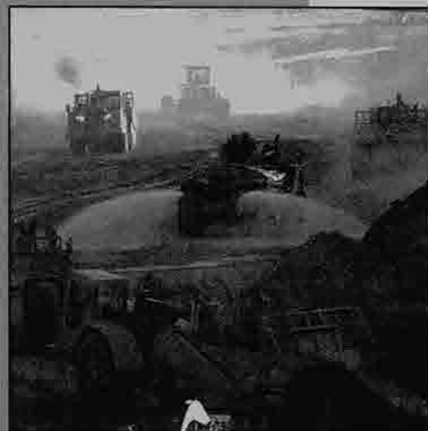
➤ Several of Ames Construction's 22 631-scrapers move into a cut at the Micron job.
