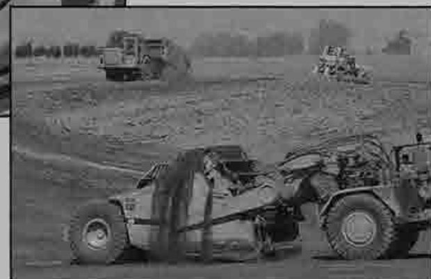
▼ An operator for American Paving fills the can at a cut on the north end of the project.
