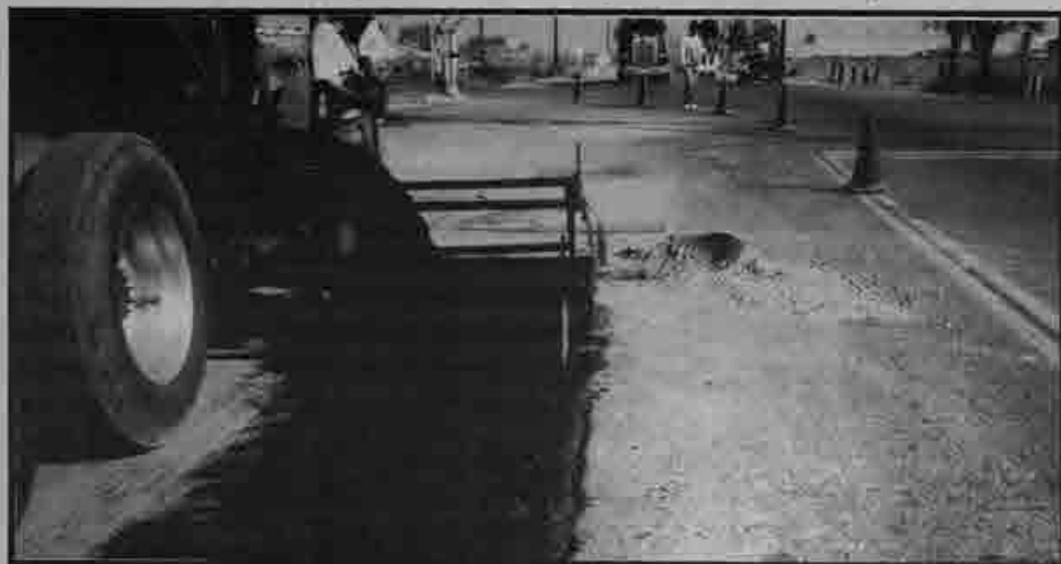
Sal Dorado's trench paver attaches to the front of a bucketless skip loader. The two rollers located on the front of the hopper rest against the tires of the dump truck. The long steel bar extending out from between the rollers connects to the truck's spreader bar. The object on the far right is the adjustable screed box.
