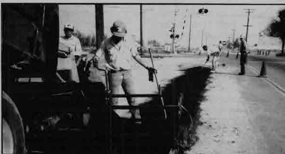
A conveyor belt moves the material out into the screed box, which can be adjusted for width and thickness.
