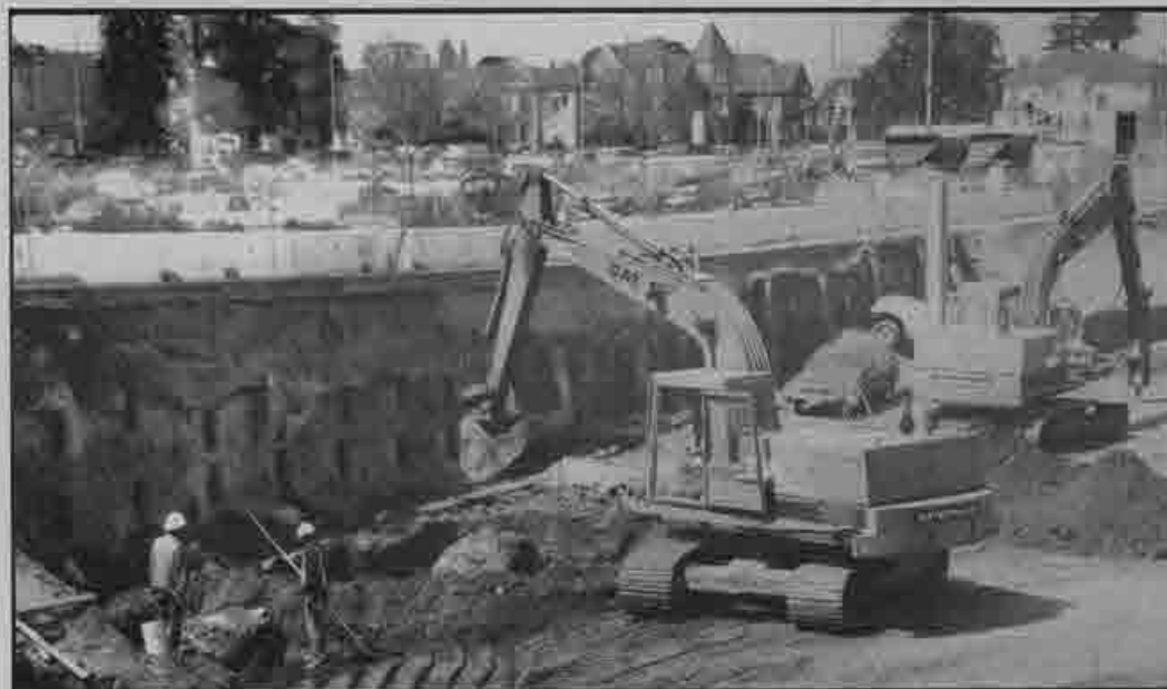
At the General Services Administration building under construction in Oakland, Local 3 operator Jack Burris breaks concrete footings using two Cat 225 excavators.
