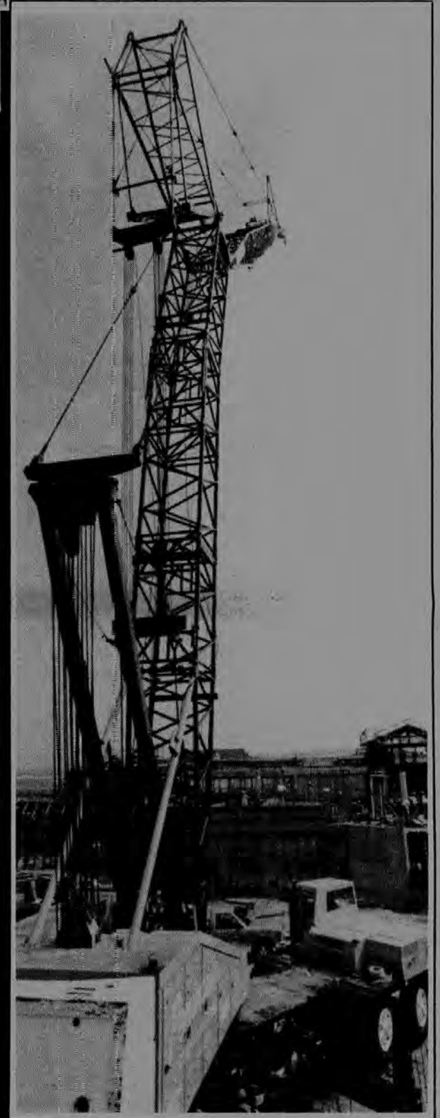
Photo at left is an aerial view of the aquarium which is currently under construction in Monterey. Pictured below is the Linkbelt crane owned by Peninsula Crane in San Jose. Featuring 70 ft. of tower with 180 ft. of boom, the 140-ton Linkbelt is the only one of its kind in California. Pictured bottom left are: Frank Chavez, apprentice; Sven Hasselberg, project superintendent; Tom Armer (back row), business agent; Billy Algers, operator; Don Luba, district representative and an unidentified worker.
