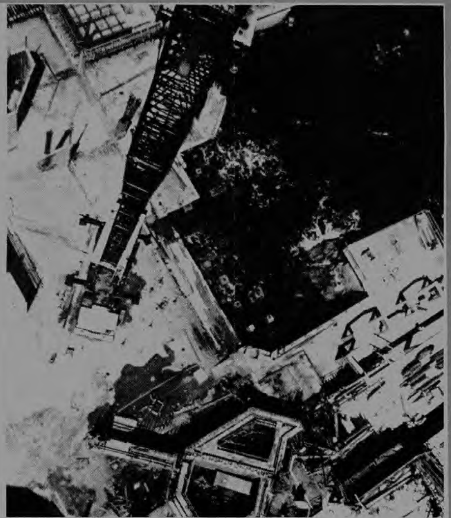
Dangling from the top of a massive 238A Linkbelt crane, a photographer for the Monterey Aquarium took this stunning shot of the $25 million Monterey Bay Aquarium project now under construction. More photos and story on page 5.
