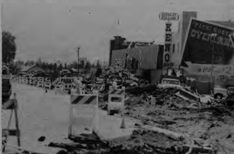
Pictured above is phase one of the B Street development project in Sparks, Nevada. Granite Construction Co. has the contract on the job. On the left is John Asquaga's Nugget and on the right is the Sparks Gold Club.
