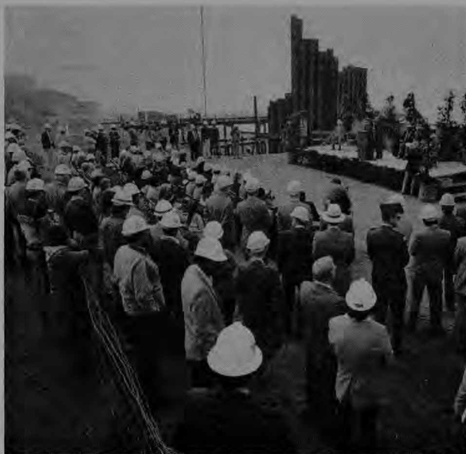
Groundbreaking ceremonies were held this month for the $165 million Ocean Beach outfall project, which was recently awarded to Morrison-Knudson of Boise, Idaho. S.F. Chronicle photo by Mike Maloney
