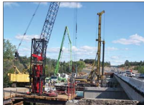
Members with Golden State Bridge drive pile, while American Concrete Placement pumps concrete on the Hwy. 44 Dana to Downtown project.
