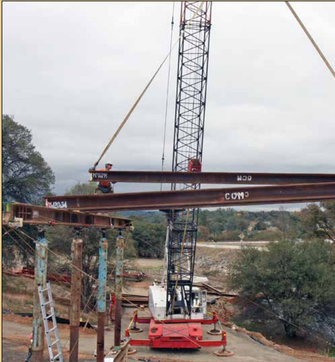
C.C. Meyers Crane Operator Mike Crowe lifts falsework for the bridge. From the northeast side of the Foothill Oaks Interchange project bridge falsework is visible. The four-lane bridge is 237 meters long and 23.7 meters wide.
