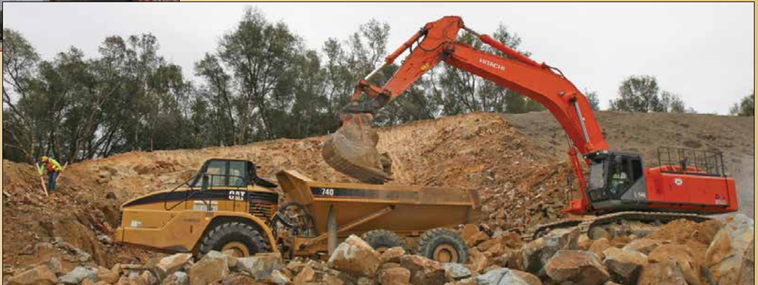
Gradesetter Dean Palmer checks grade while Excavator Operator Matt Barker works with Articulated Dump Truck Operator Brian Foucek to dig footings for the Foothill Oaks Interchange in District 80.
