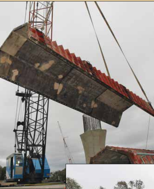
Crane Operator Cynthia Cruz places the forms for the Foothill Oaks Interchange pillars on a truck to be loaded away.
