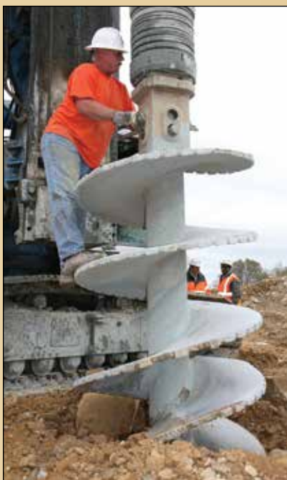
Working for Malcolm, Oiler Russ Starr readies the drill as Operator Bill Leigh prepares to drill 37-feet down in dry-packed earth. The holes will be used for cages to support the Foothill Oaks Boulevard Interchange.
