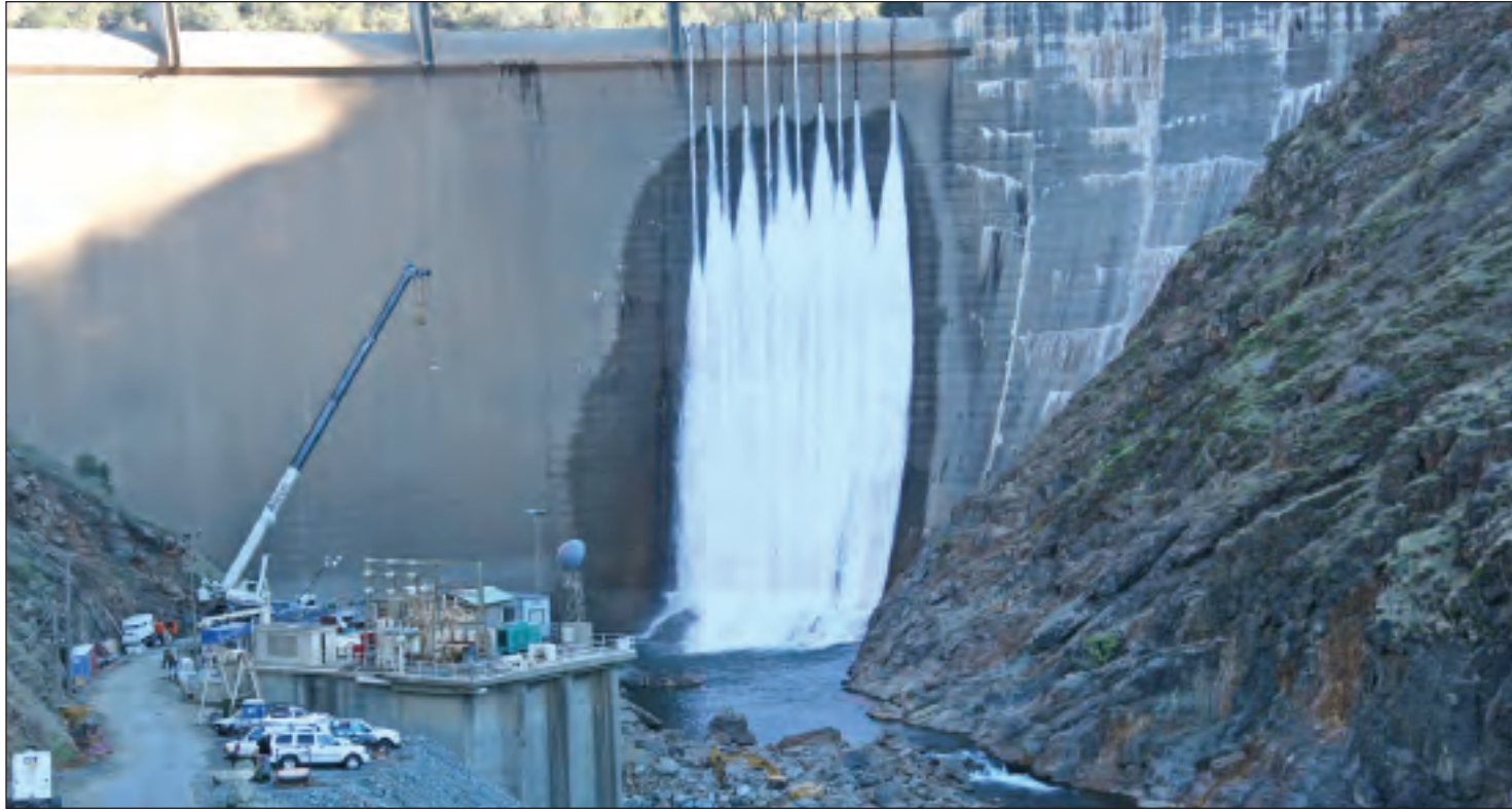
Built in 1941, the Englebright Dam maintains the 70,000 acre-feet of Englebright Lake. The temporary 60,000-pound valves pictured here siphon continuous water to the Yuba River below.
