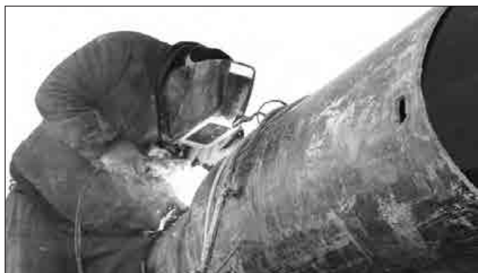
Local 3 member Salvador Vargas welds a section of pipeline before it is lowered into the well.
