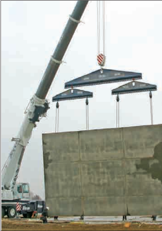
Local 3 Operator Robert Wilkes Sr. uses a 265-ton Liebherr Crane to set a section of prefab siding for a retail store in Yuba City. The crane is owned by Bigge Crane.
