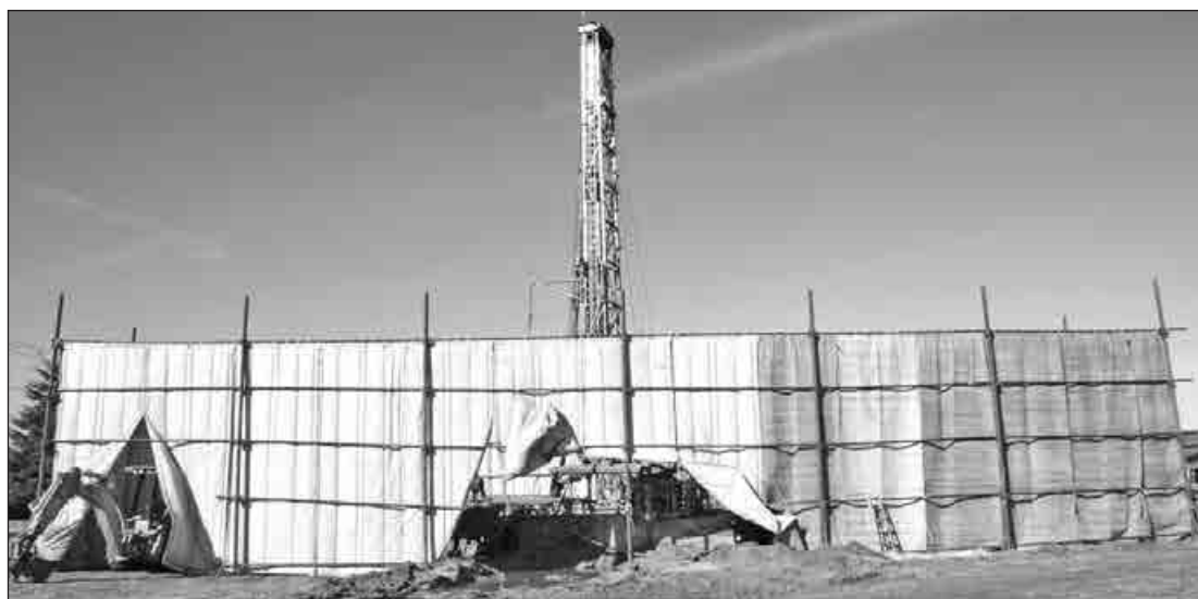
This sound curtain is used on the Maggiore Bros. jobsite in Salinas to lower noise levels from 100 to 60 decibels.
