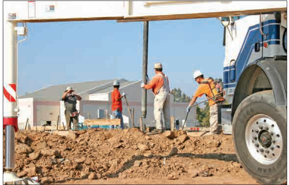
Crew members pour concrete for the footings of a church in Fresno.
