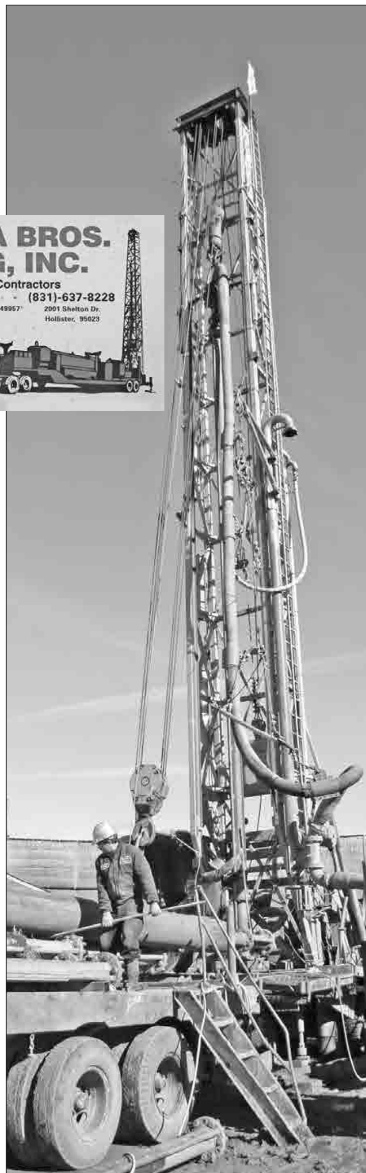
Maggiore Bros. uses this drilling rig to dig a 400-foot-deep water well in Salinas.
