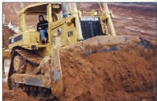
Operator David Workman works for Garrett Construction on the Clovis jobsite.
