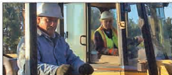
At the controls are Local 3 members Matt Muehlenbeck (foreground) and David Jimenez.
