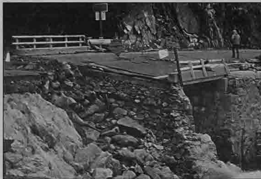
Bridge takes a beating: This damaged bridge and approach on Hwy. 49 between Camptonville and Downieville in Sierra County will require extensive repairs.
