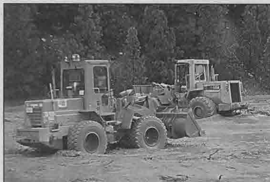
Pushin' mud: A Caltrans loader teams with one of J.F. Shea's loaders to remove mud on I-5 at Sweetbrier.
