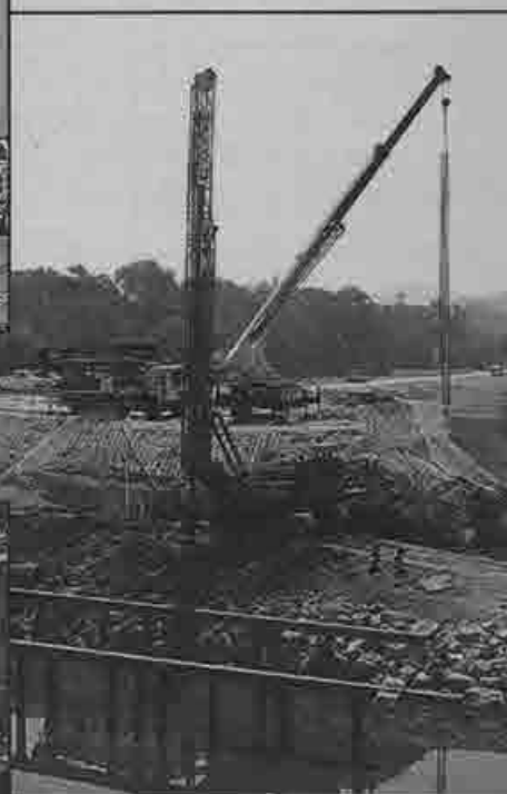
Pile driving: Malcolm Drilling driving piles for the new bridge over Cache Creek, with support from Berkeley Concrete Pumping
