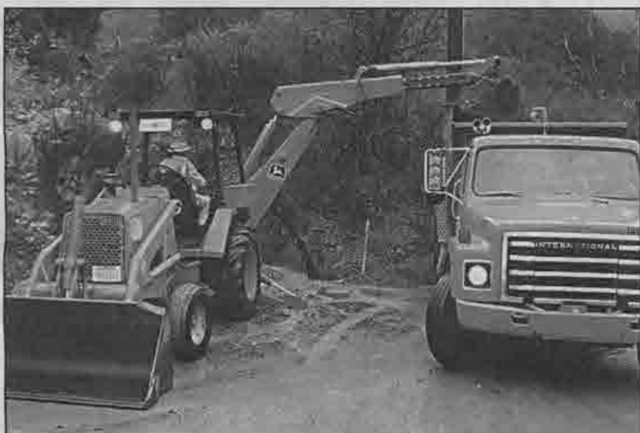
Mud's a flyin': Backhoe operator Larry Mears cleans a drainage culvert on Niles Canyon Road.
