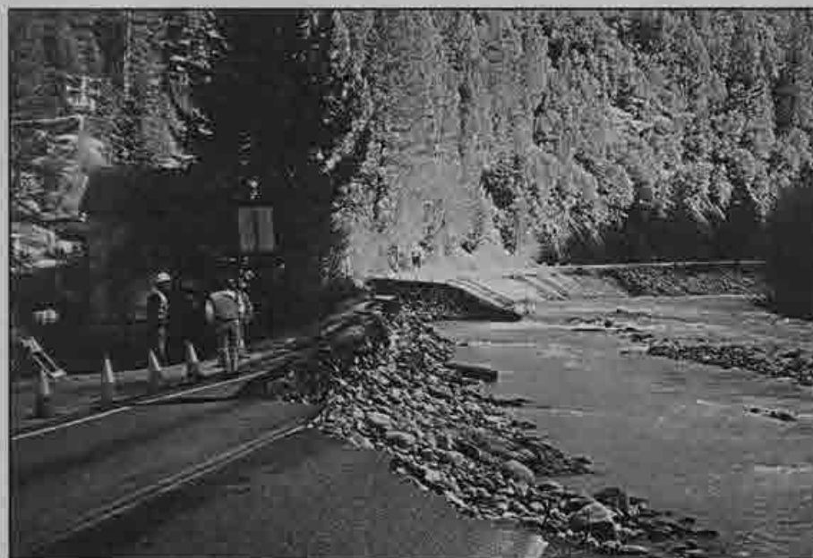
Highway gives way: A washout on Highway 49 near Downieville.
