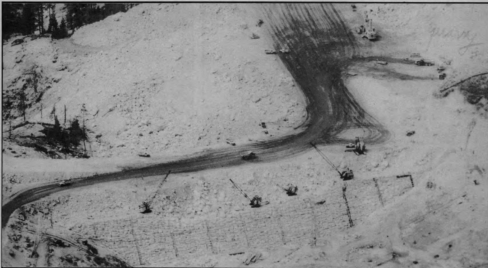
Above: Crane's place rock on the face of Bear River Dam between 1951-1954.
