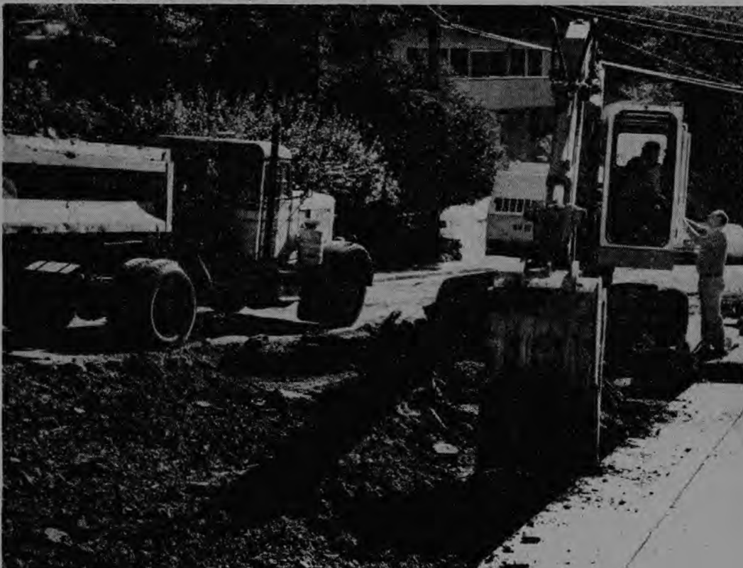
Local 3 backhoe operator breaks asphalt off street that was undermined by flood water in San Rafael.
