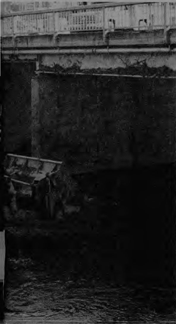
Granite Construction operator Robert Brown digs a channel (left) near the abutment of the Soquel Bridge so engineers can determine the extent of the damage. Business Rep. Jack Jackson, who was on the scene during the storm helping with emergency problems, said that during the cleanup at the bridge, a giant chunk of redwood weighing several tons was dug out of the
