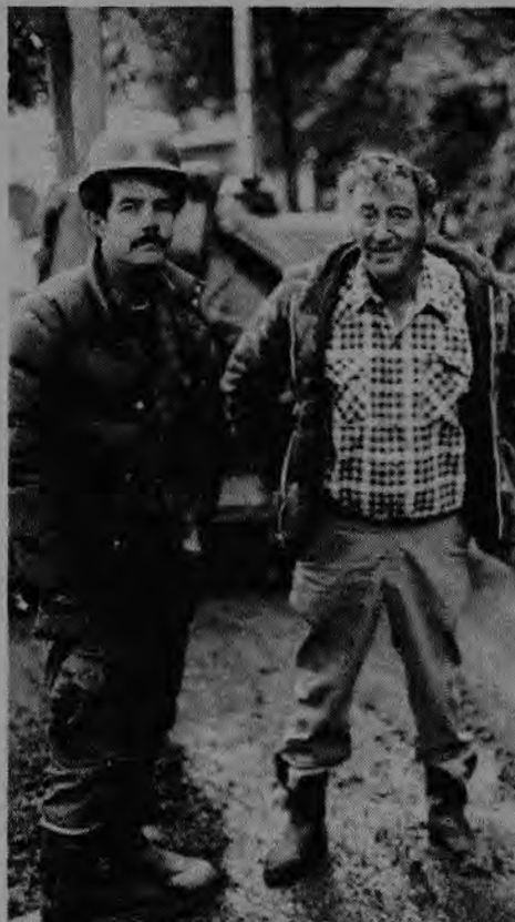
Local 3 members Kirby Bobo and Harry Merz working at Hurricane Canyon slide in Sausalito.
