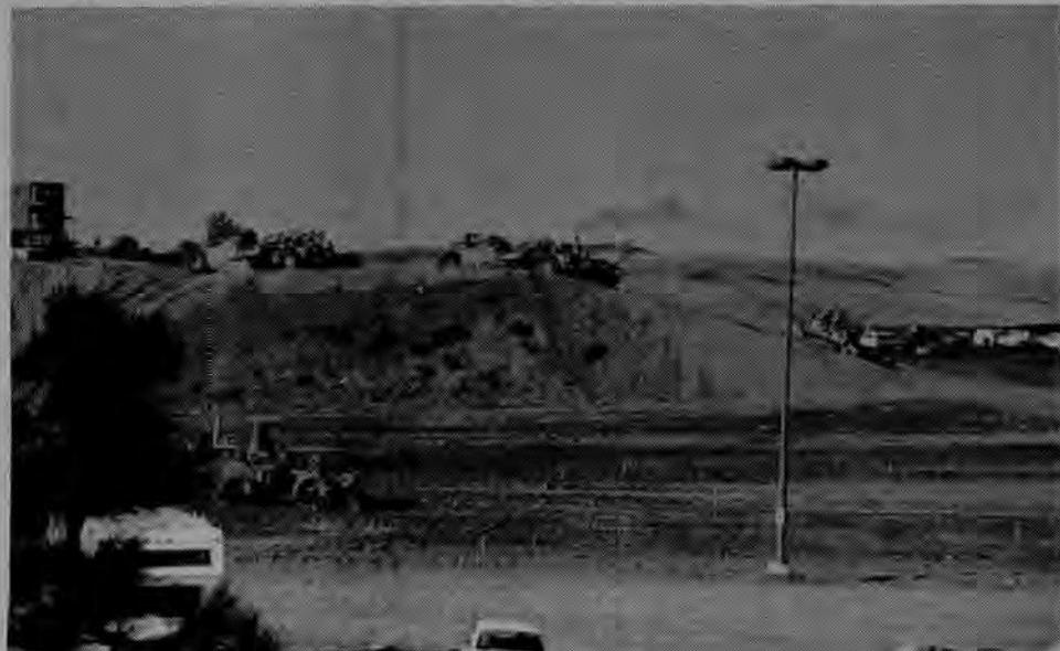
Pictured above is the site work being done on the sports pavilion at the University of Nevada, Reno.
