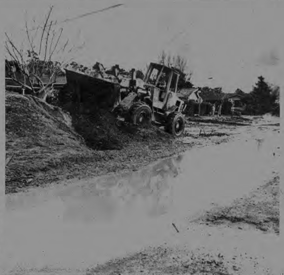
A Local 3 member working for Ghilotti Construction moves mud and debris off the street to clear a way for emergency vehicles in San Rafael's Glenwood area, which was hit badly by the storm.
