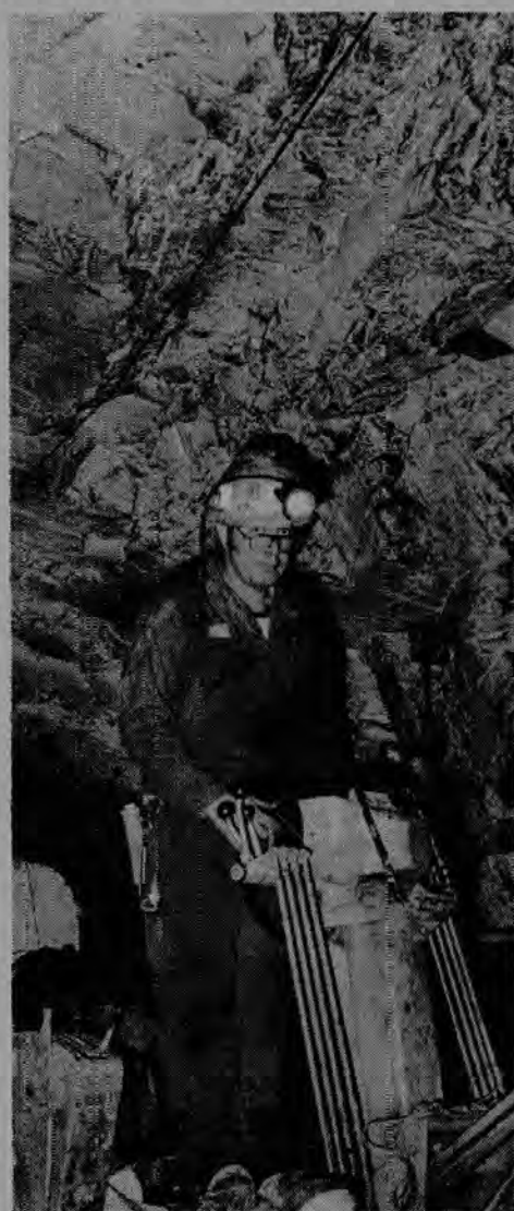
Local 3 member George Young runs a motor patrol 4,000 feet underground, cleaning up drift in the narrow work tunnels.
