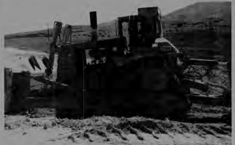
Local 3 member Dennis Gallagher mans a CAT D-10 on Jack B. Parson's I-80 job at Wendover.
