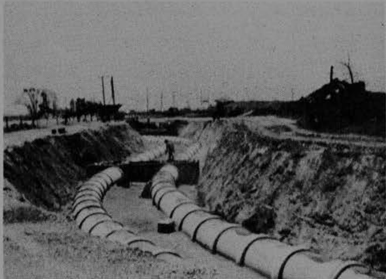
Working behind the backhoe, a conveyor spreads rock on the Super Sewer job in the East Bay (top photo). In the center photo, the Drott is waiting to lift a section of the sewer pipe into place. Bottom photo depicts the two 39-inch pipelines making a fancy curve.
