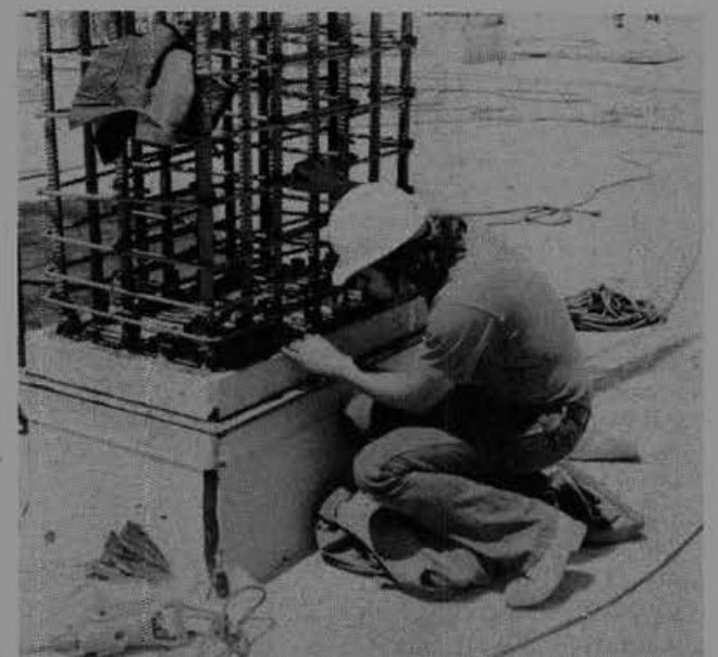
N.D.T. technician Wayne Young conducts a visual inspection of rebar on the Pacific Telephone Co. addition in Santa Rosa.
