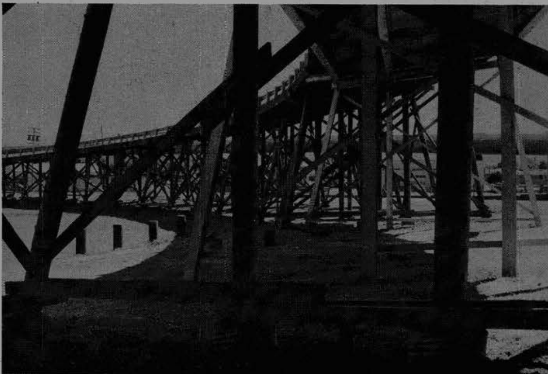
PICTURED ABOVE is part of the temporary wood piling supporting the Rt 92/101 interchange.
