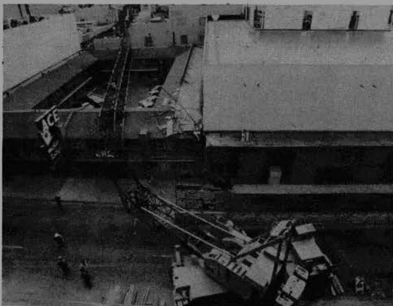
A 280-FOOT AMERICAN TRUCK BOOM wrapped itself around a Reno motel like spaghetti recently, when a gust of wind apparently caused the untied demolition ball to throw the boom off balance. Although there was considerable property damage no injuries were sustained from the accident.
