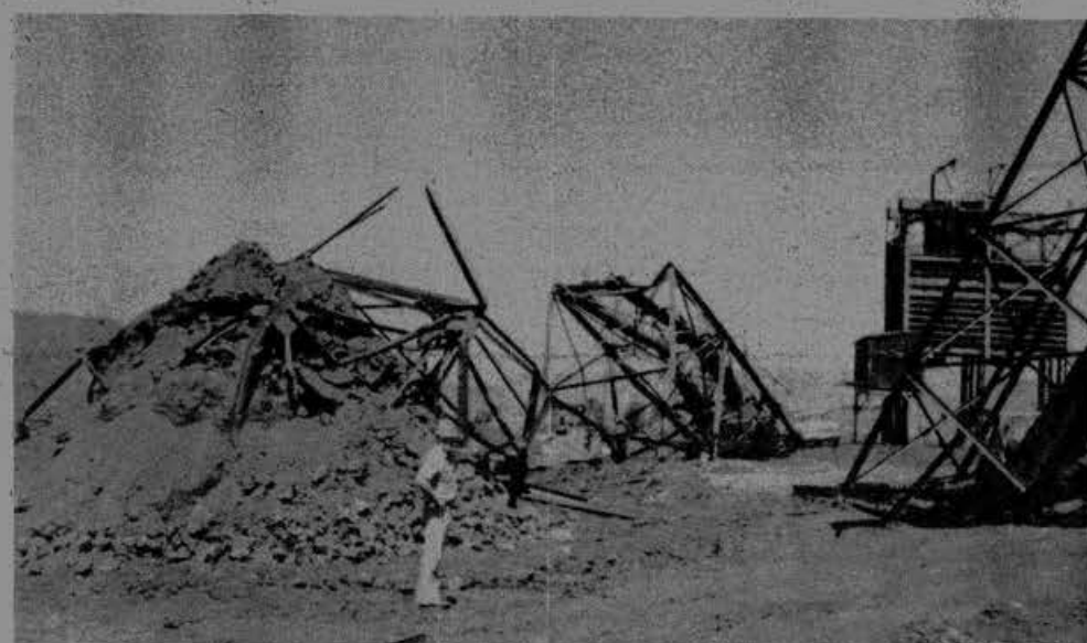
Pictured above is the conveyor system that collapsed at Utah International's iron mine near Cedar City.
