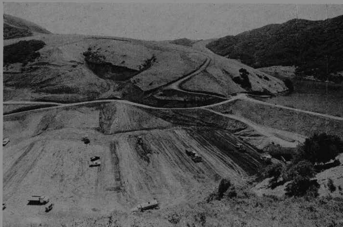
Engineers News Photo PICTURED ABOVE is a top side view of the new Soulajule dam in Marin County. To the right is the old dam. At bottom left, workers construct the 48-inch outlet line that will transport water to the pump house. The scraper pictured below looks like a head without a body—actually the driver was simply making a sharp left turn. Local 3 member Larry Eaton mans the scraper pictured bottom right.
