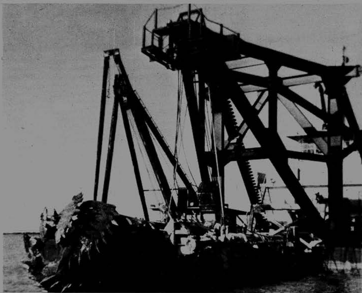
THE EXPOSED CUTTERHEAD of the 36-inch dredge Hydro Pacific is seen above.
