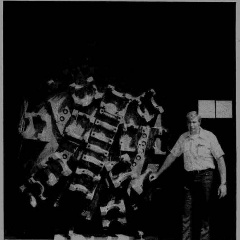
Marysville Business Rep. Dan Mostats stands next to the 12-foot-high Perini mole, which was used recently at Oroville. The cutting heads have been removed in this picture.
