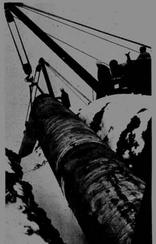
Workmen lower a 36-inch natural gas pipe on Flathead Ridge, British Columbia at an elevation of 7,000 feet.
