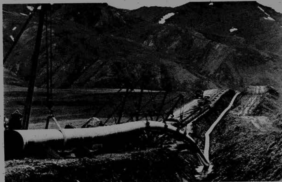
A section of 48-inch pipeline is lowered into a ditch by sideboom tractors in the Brooks Mountain Range, 175 miles south of Prudhoe Bay. Nearly half of the 800-mile pipeline is buried.
