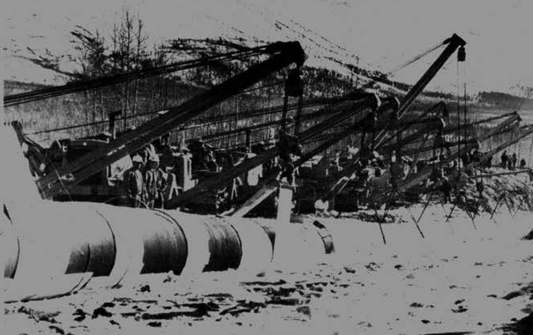
The pipeline installation at the Tosina River in 1975 was the first of some 30 miles of river crossings along the 800-mile long trans Alaska pipeline.
