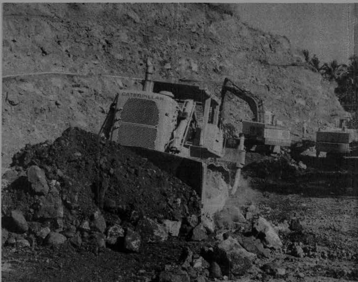
Albert Chiappetta cuts away part of the hillside with his D-9 Dozer, while brothers Patrick Cabral and John Yu operate backhoes in the background. The project is a portion of a road that is being constructed near Hawaii Loa.
