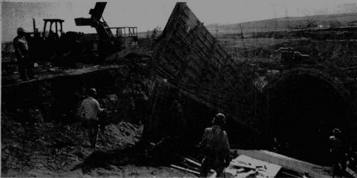
WORKERS SET a concrete form (above) onto the largest siphon on Reach 6 of the canal.
