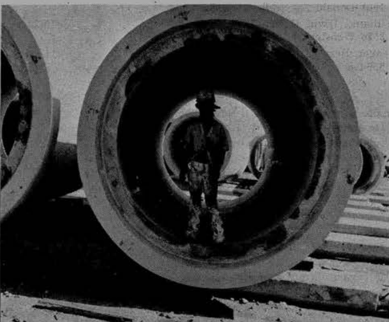
BIG IS THE WORD for the 12-yard loader on which Herbert "Red" Denning is standing in the top photo and the 84-inch pipe which surrounds apprentice Samuel Wong in the bottom photo. Both men are working on the Honolulu outfall line project.
