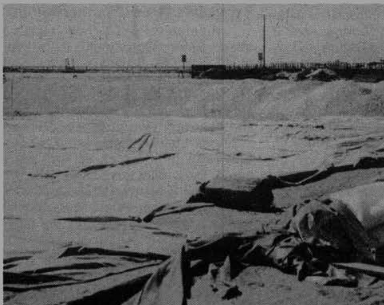
Pictured top are the nylon and polyester rolls being used to blanket the sawdust. Next picture shows worksite being prepared with Dumbarton Bridge construction in background. Pictured right is portion of project with nylon blankets rolled out.
