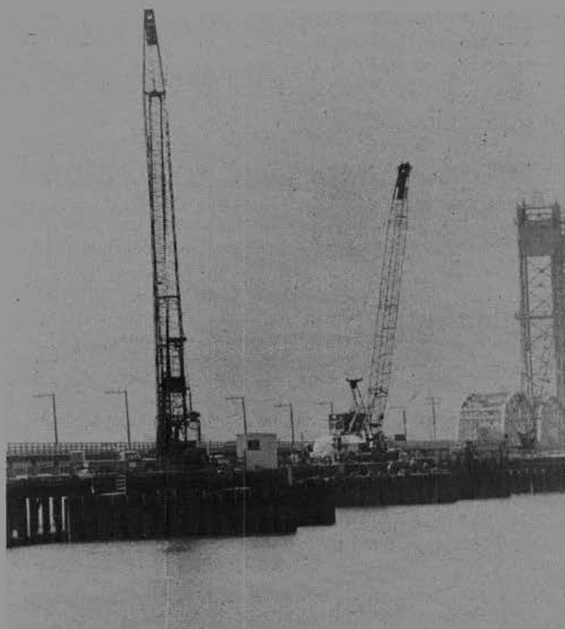
Workers construct access trestle on Dumbarton Bridge
