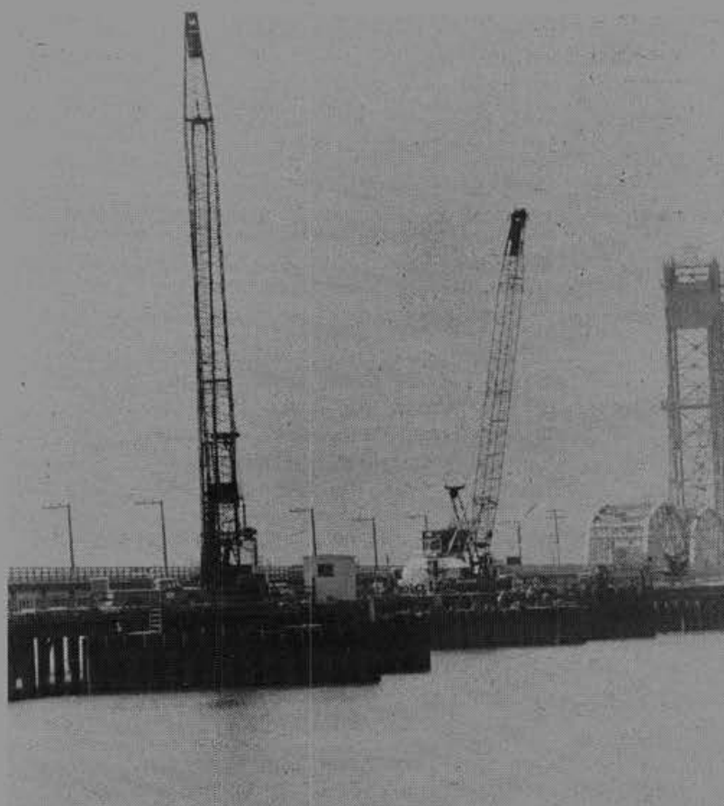
Workers construct access trestle on Dumbarton Bridge
