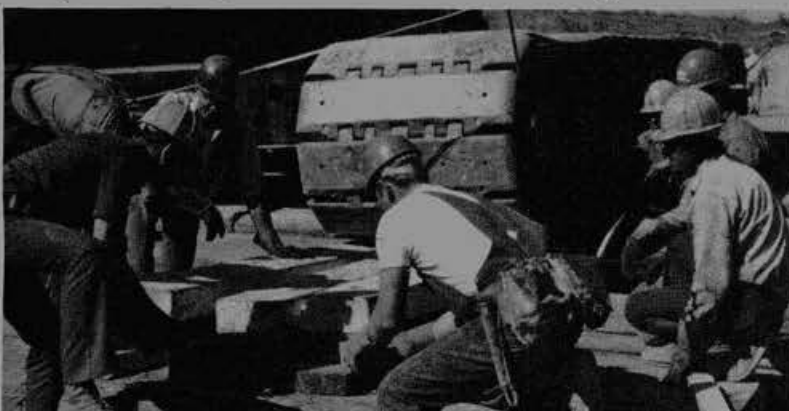
The crane is set back down and iron workers insert extra pads beneath the Manitowoc 4,100.
