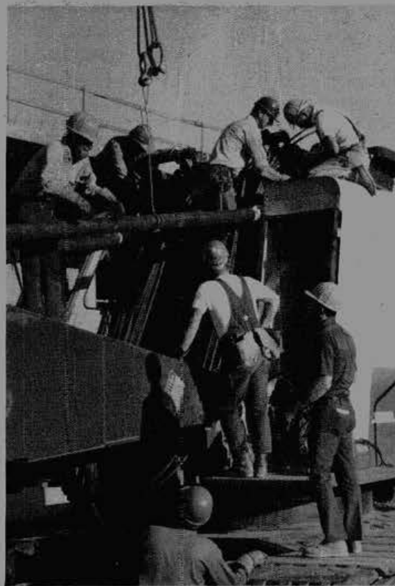
LIFTING A CRANE requires a lot of preparation. Above, iron workers strip the boom off the Manitowoc 4,000 and position pads on the span where the crane will be placed for setting the heavy steel spans across the slough.
