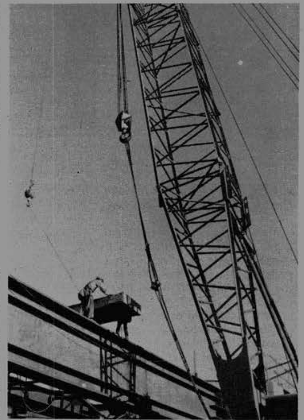
position pads on the span where the crane will be placed for setting the heavy steel spans across the slough.
