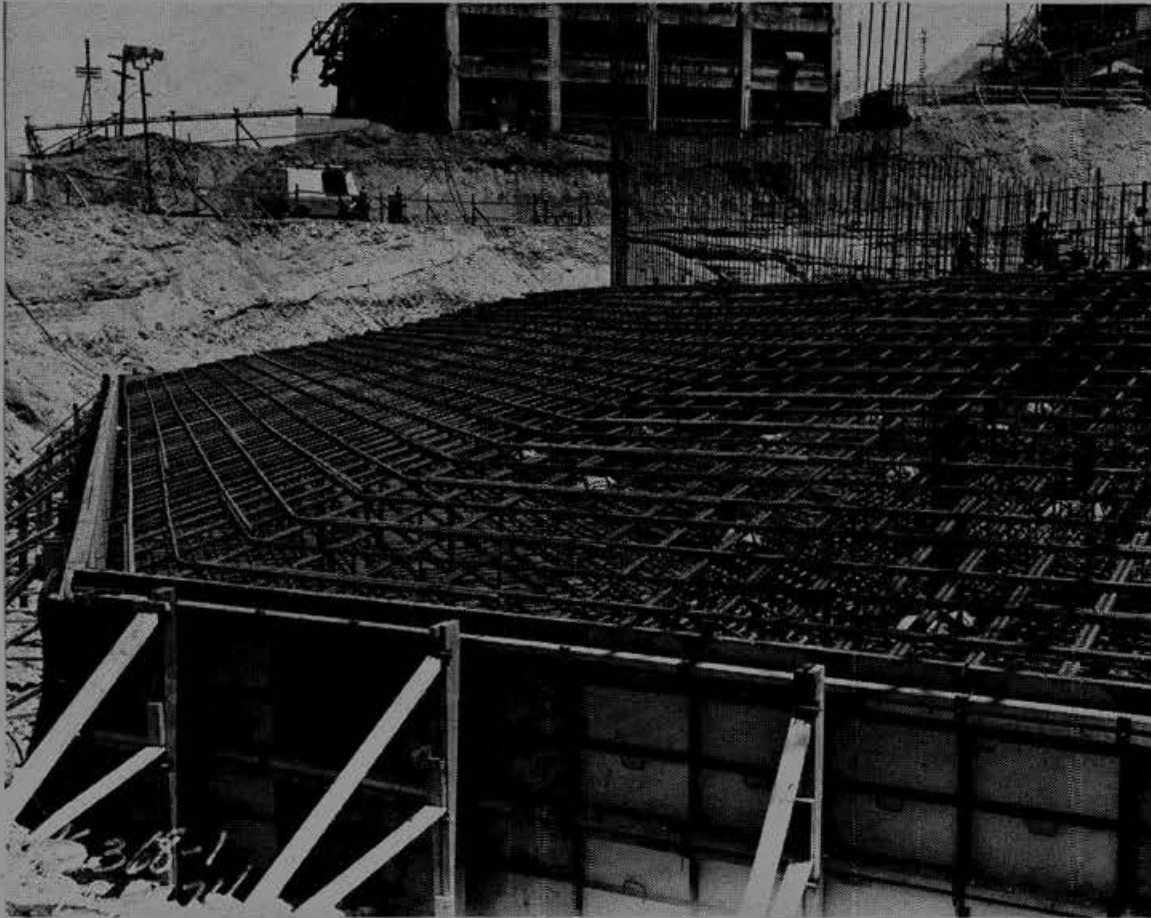
THE BASE of Kennecott Copper's projected 1,200-foot smelter stack began with the form shown above. Two days of continuous pouring were needed to fill the form.
