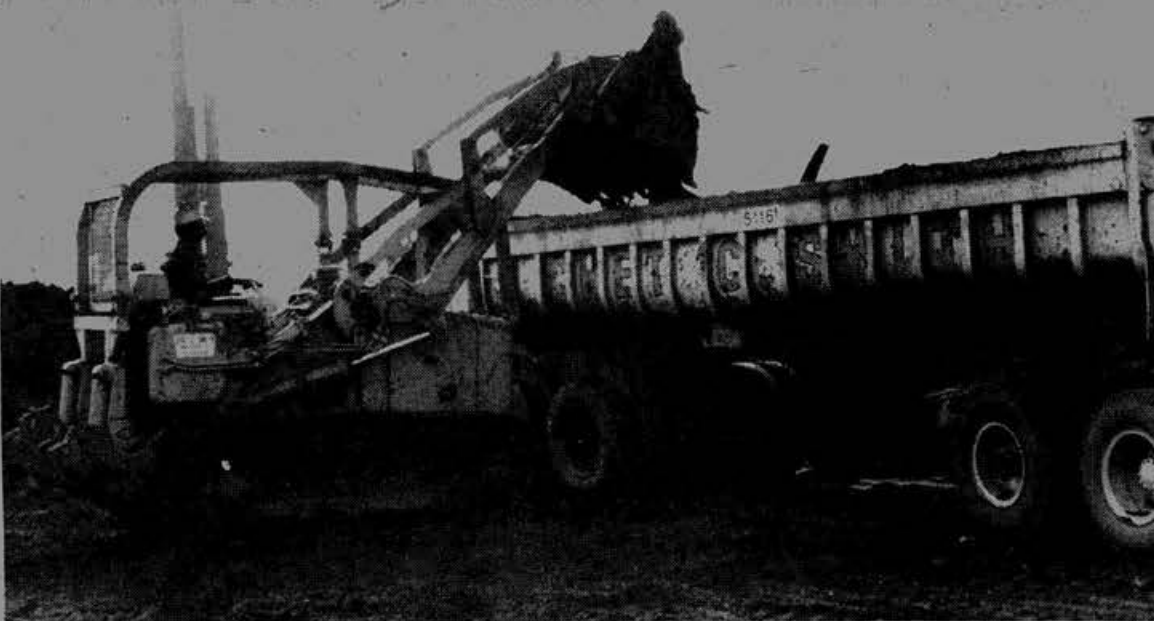
THE FIRST job of the billion dollar San Francisco sewer project is now underway. The contract calls for construction of a large pump station that will pump sewage from the eastern shoreline to the south treatment plant.
