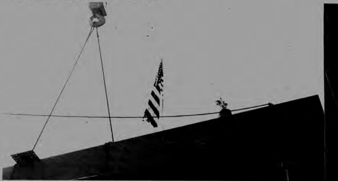
TRADITIONAL EVERGREEN GOOD LUCK tree (middle photo) was placed on the newly completed 2,428-foot span along with the American flag which once flew above the Capitol. The flag was
