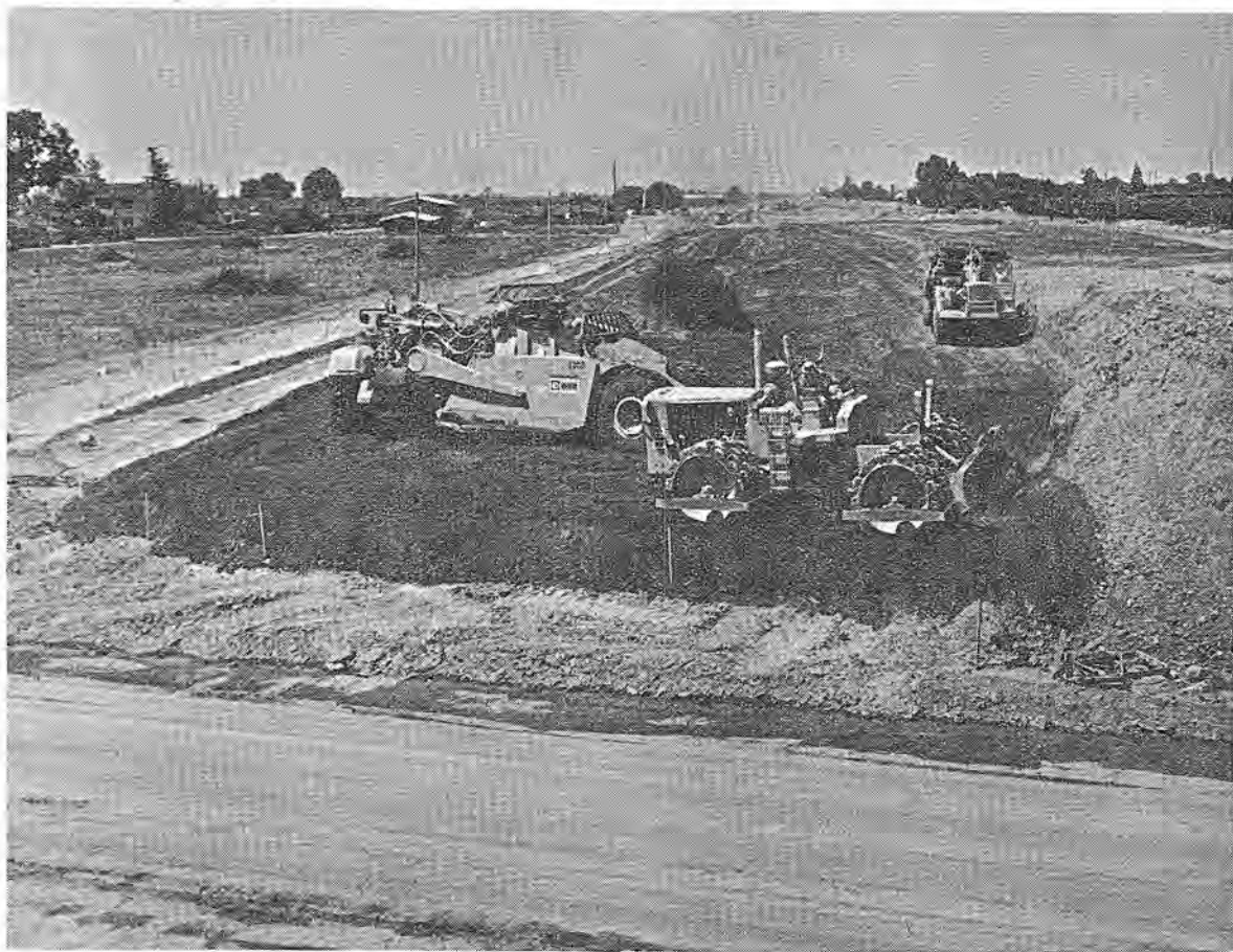
BUTTE HOUSE ROAD in Yuba City (at bottom of photograph) is open to traffic between Yuba City and the Tierra Buena area while 600,000 cubic yards of fill are relocated at Onstott and Butte
