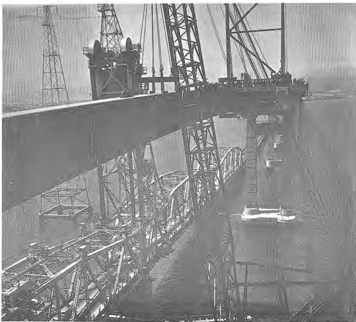
FINAL LINK in the $70 million San Mateo-Hayward Bridge goes into place. The two girders, longest and heaviest on the bridge, weigh-in at 520-ton and are 380-ft. long. E. R. Foley, chief engineer,
