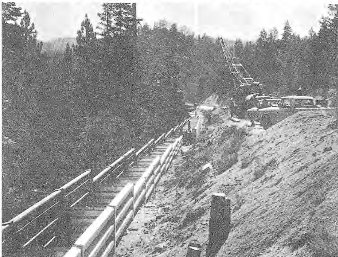
Because of a high backslope and soft materials, bin-type retaining walls had to be used on the Tahoe highway project. Cost of the bins was estimated in excess of $200,000.
