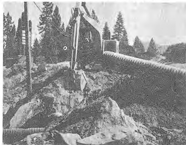
Arduous task of setting culvert in rocky ground was just one of the problems encountered in road construction.
