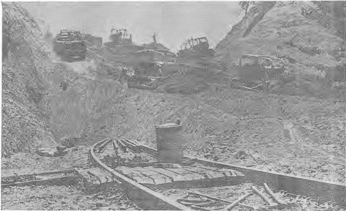
Rail service 10 miles north of Ukiah was halted when tunnel burned, but 12 Cats bore down on the job, and within 48 hours, had rail service restored, but without burned out tunnel.
