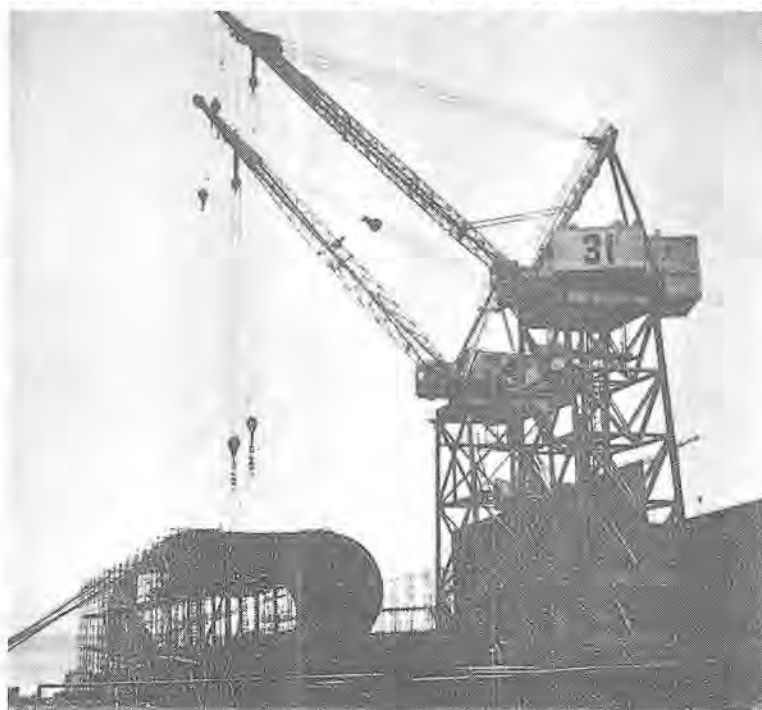
Two 80-ton cranes lift tube section of BART system, being built at Bethlehem Shipyards. Tube Segment is 300 feet long.
